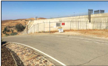
Friant Dam is triangle shaped and about a mile long at the top.
