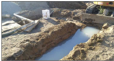
The machine dug deeper and deeper, until they found water. When the Muller family first saw the water they were excited!
